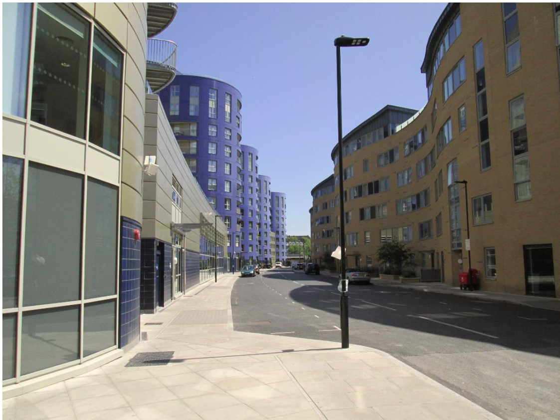
View looking east along Queensland Road.
